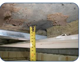
CB-RR-50 with C Channel, fiberglass and gypsum board
